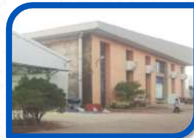
Injection Moulding + Assembly (75000 sq. ft.) Goa
