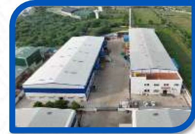
Unit 4 - EPS Moulding + Assembly (100,000 sq. ft.) Chennai
